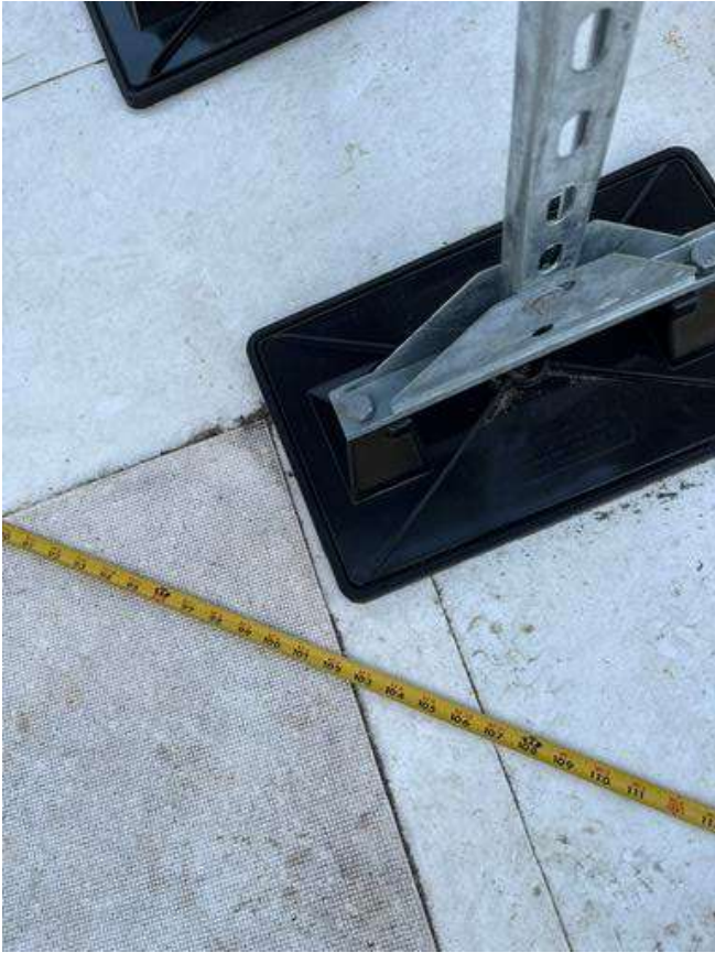
Duct Support Spacing
